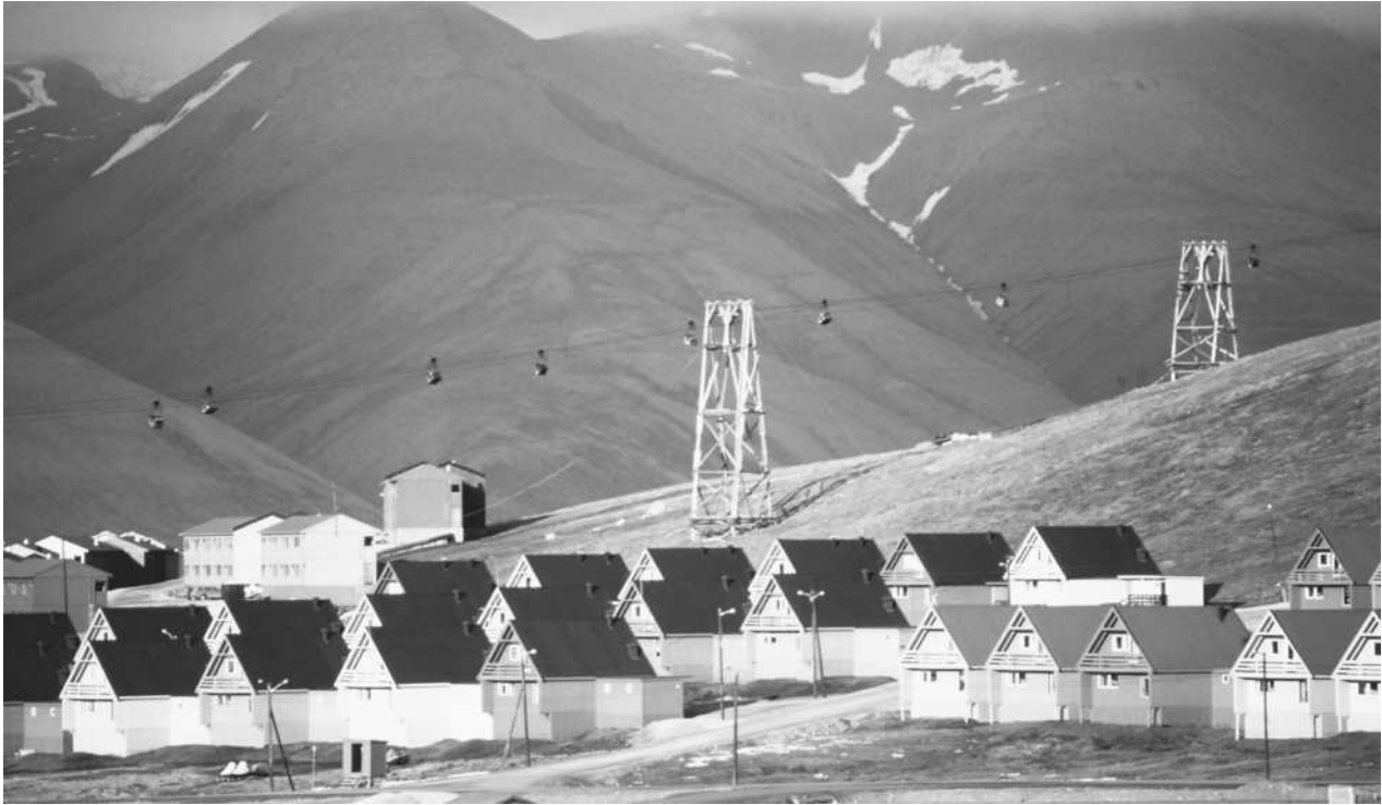
A collection of houses built for coal miners and painted colorful tones to reduce suicide rates in the long, dark winters of Spitsbergen.
